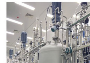
Intelligent pressure regulating valve system
